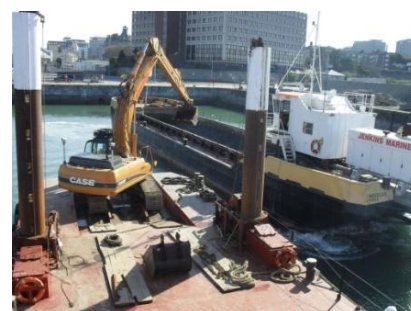
Dredging underway at Millbay
